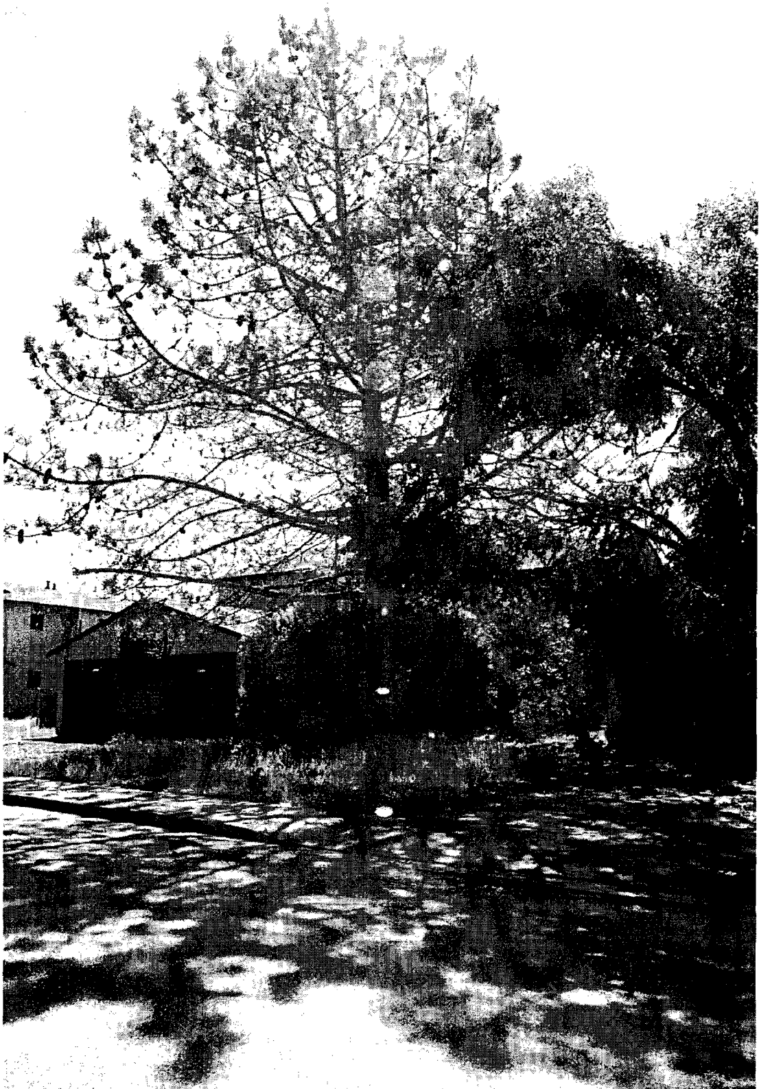
Roots are lifting street
